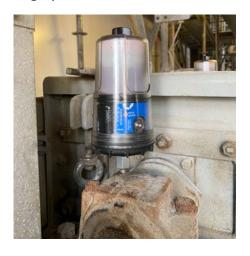
Single point lubricators apply lubricant to a single lubrication point. They are most commonly used to lubricate bearings, but can also be used to lubricate pumps, electric motors, fans, chains, linear guides, open gears and conveyors, amongst other applications.
